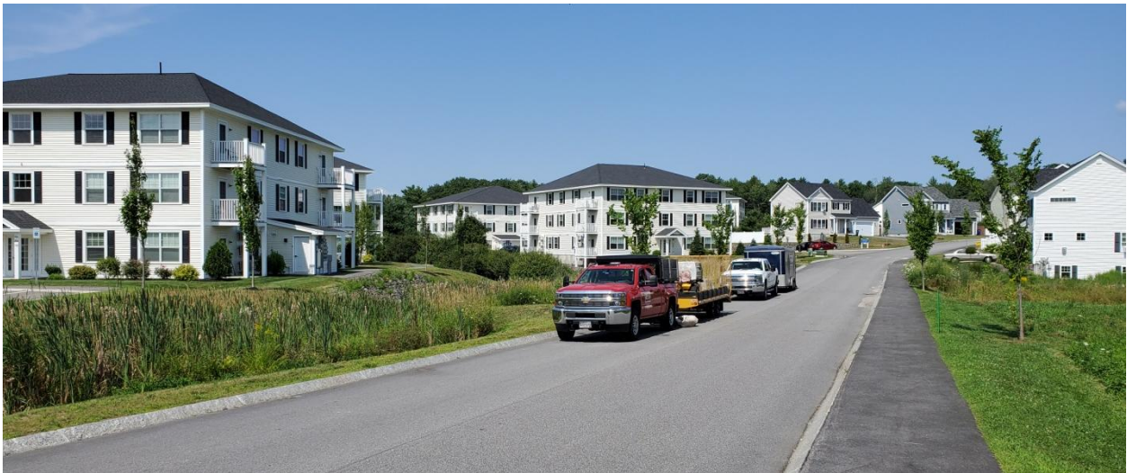
Figure 2 - Blue Spruce Subdivision, Westbrook. Multi-family buildings with single-family in background.
