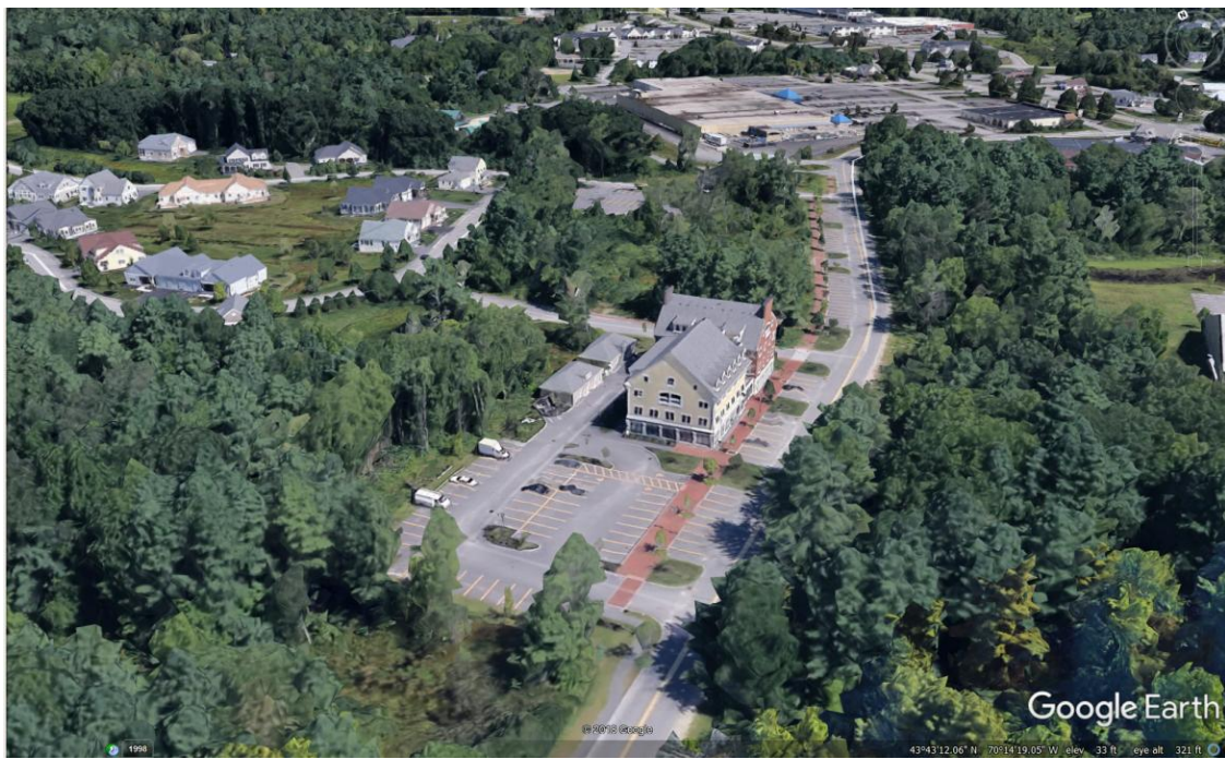
Figure 9 - Tidewater, Falmouth. Offices on floors 1 & 2, residential above.
