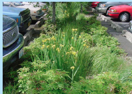
Example of parking lot stormwater treatment.
